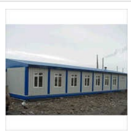
Prefabricated Labour Hutment
