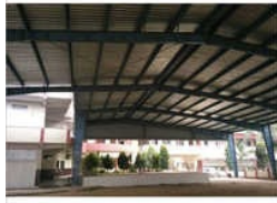
Pre Engineered Building Structure
